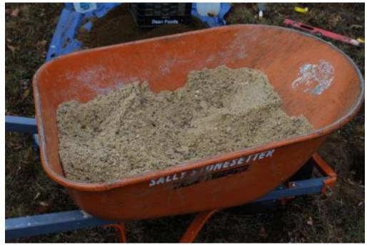
Mix pea gravel with sand Use masonry sand, not play sand which has been washed and can cause staining
