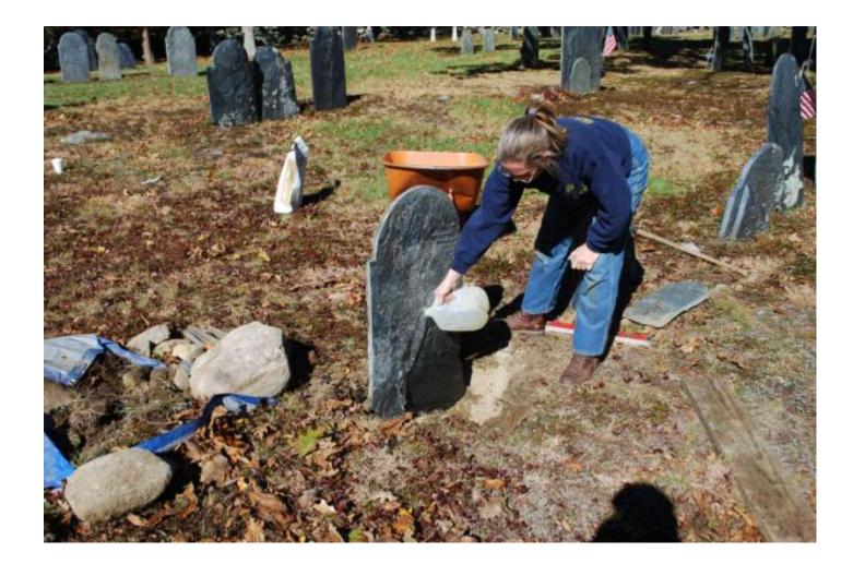
Use water to help compact the sand mix and soil Continue to tamp down and fill around stone Check stone is level as you back fill the site
