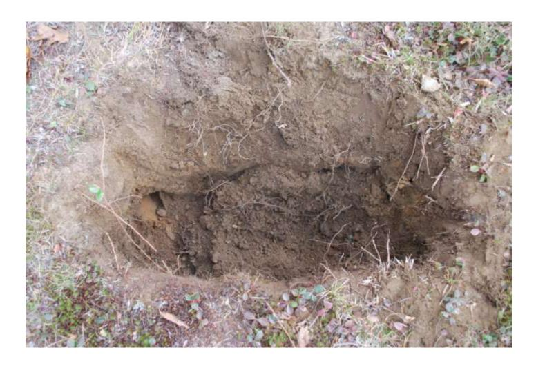
Prepare the hole which should be slightly wider than the stone and deep enough for one/third of the stone to be below grade Remove large stones and roots from the hole
