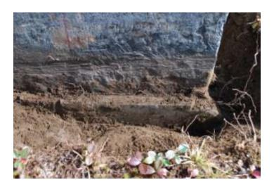
Start to careful remove soil around the bottom of the stone Wear gloves and watch for broken glass in front of the stone.
