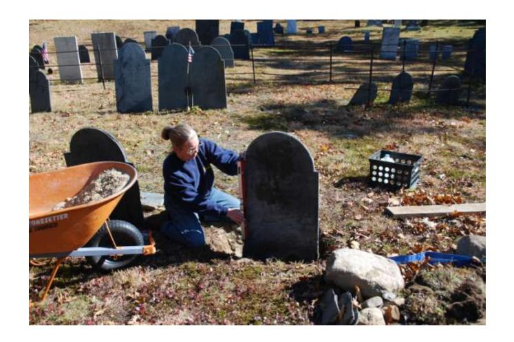
Set stone and check with a level, front to back and side to side
