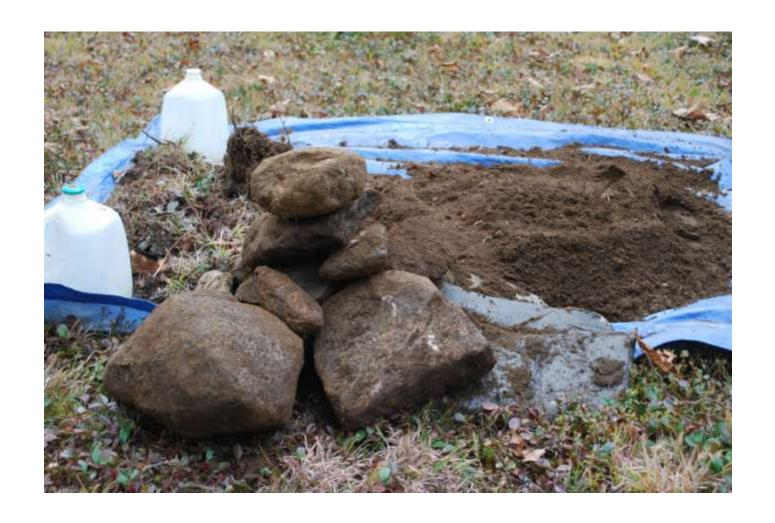
Remove all large rocks from the site Large rocks can place pressure on the gravestone and move it during the freeze/thaw cycle
